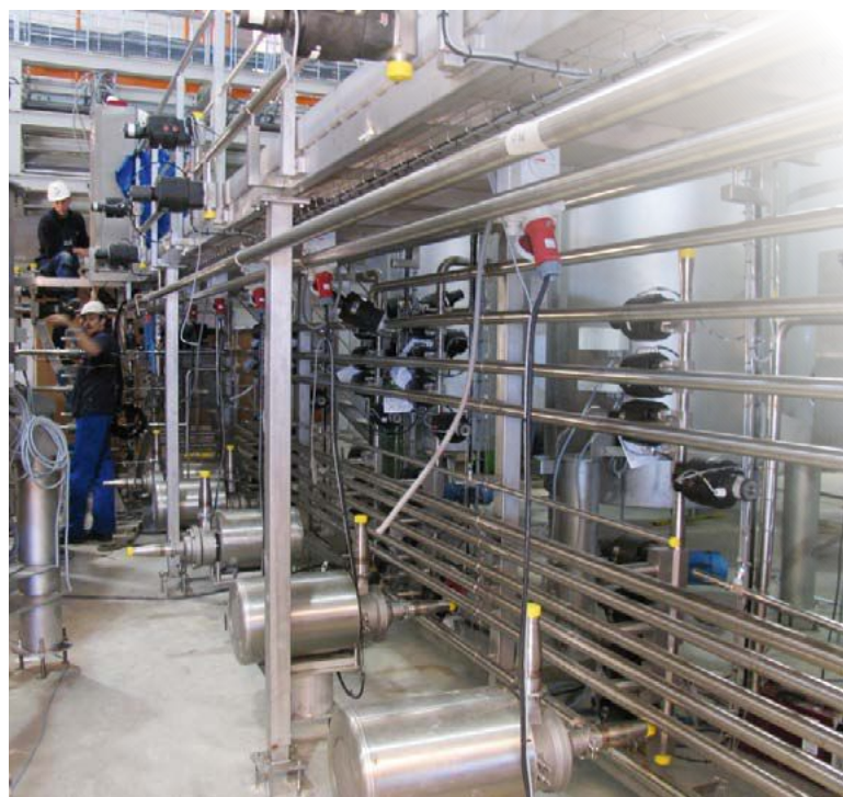
Xendo Static SMB XPure-S during construction work
